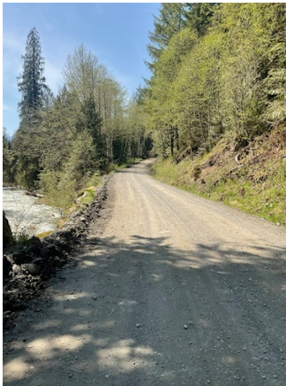
From town approach, no barrier.
